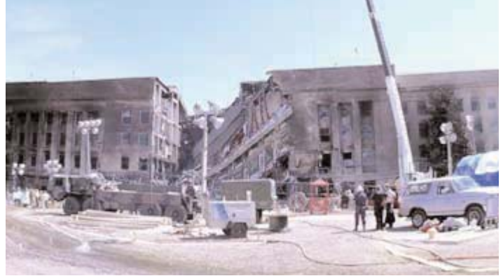
Damage at Pentagon.
